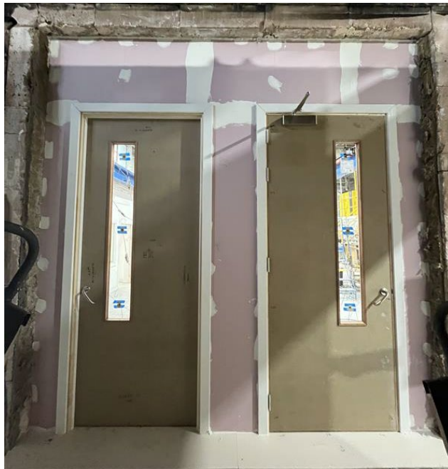
Figure 16 – The exposed surface of the test construction prior to commencement of the test
