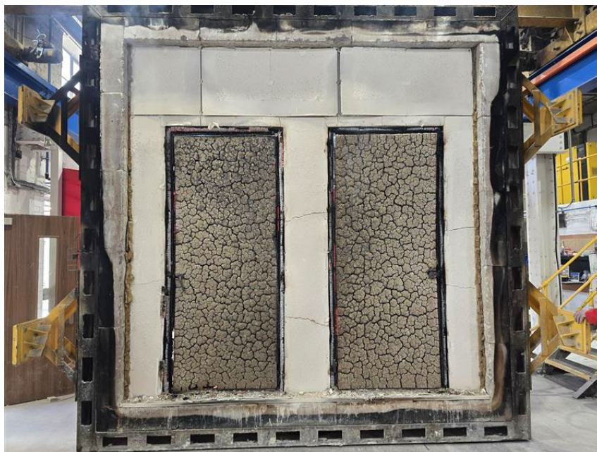
Figure 24 - The exposed surface of the test construction after the test was discontinued
